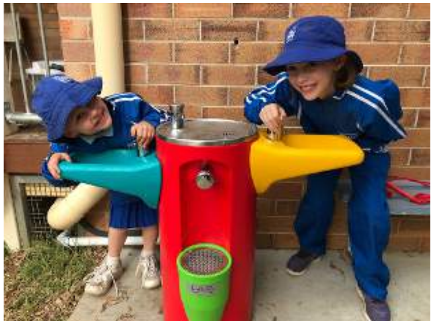
Christina and Ella using the new bubbler. The bubbler has a filter and chiller, three water spigots and a place to refill water bottles.
